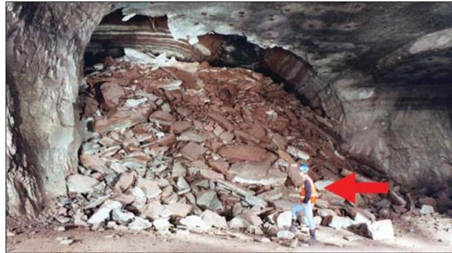
*Figure 1. Massive roof fall demonstrates some of the perils in underground working conditions. Mine inspector shows the scale of the problem. (Courtesy from MSHA).*
