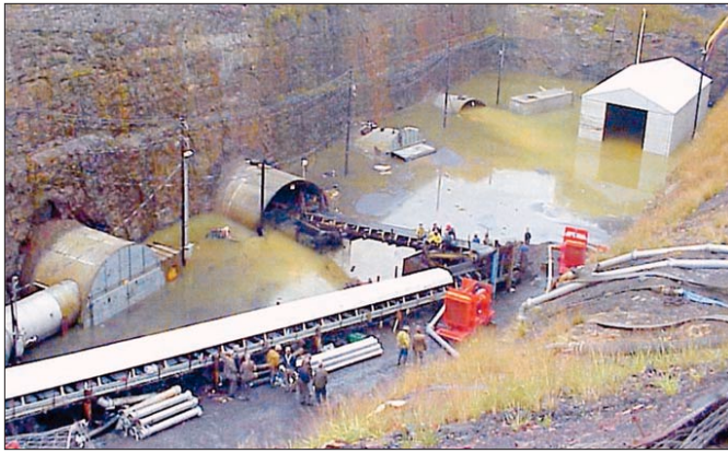
Figure 4. Flooded entrance to QueCreek Mine indicates the severity of the problem. Large capacity pumps (orange) were used to quickly drain the water before trapped miners were safely rescued.
